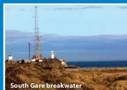
South Gare breakwater
