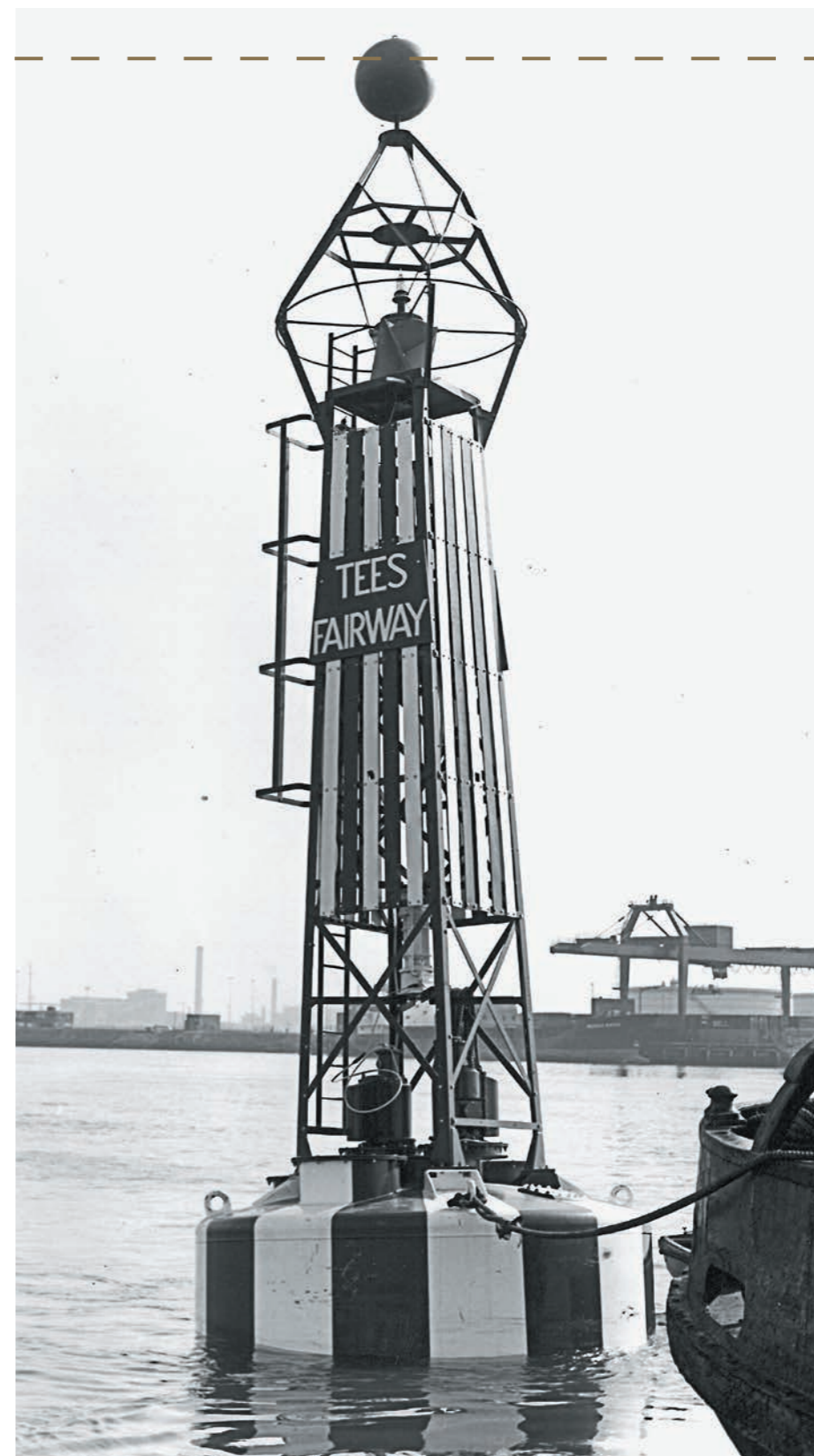
New 14-tonne Fairway Buoy. The world's largest navigational buoy, April 1982
