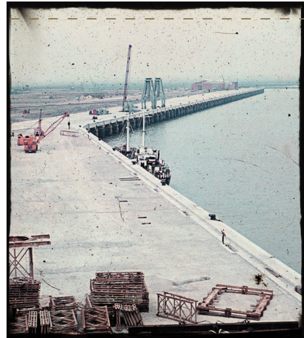
Construction of No. 1 Quay, Tees Dock, 1963
